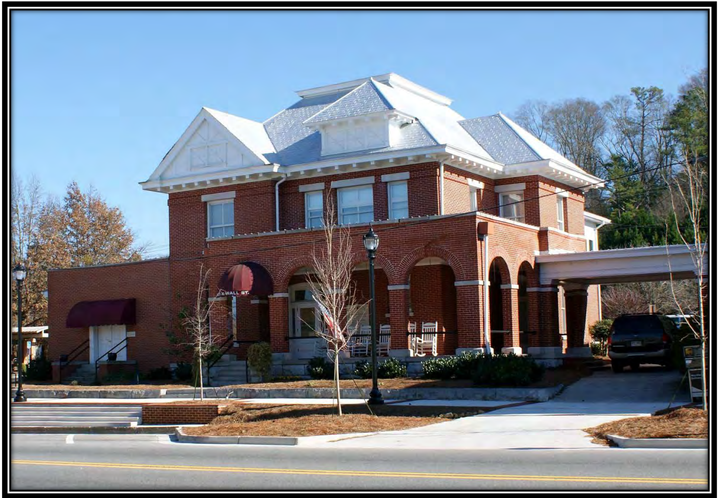
Gordon County Administration Building
