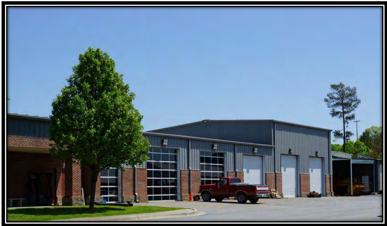
Gordon County Fleet Management Facility
