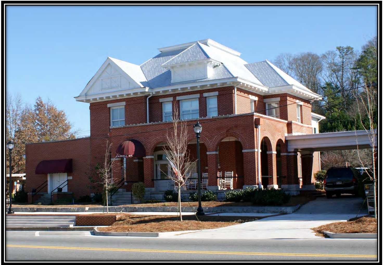
Gordon County Administration Building
