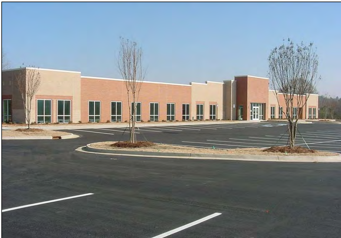
New Gordon County DFACS Building
