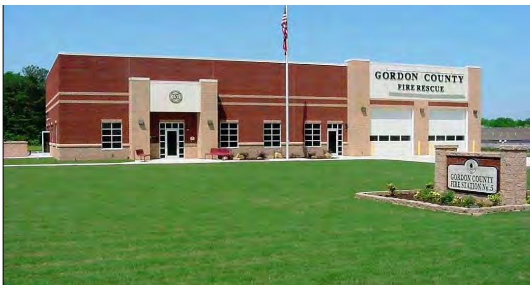
Gordon County Fire Station in Resaca
