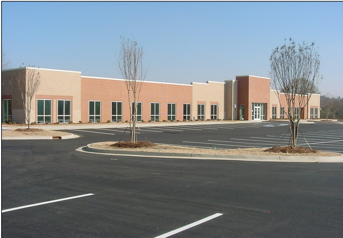
New Gordon County DFACS Building
